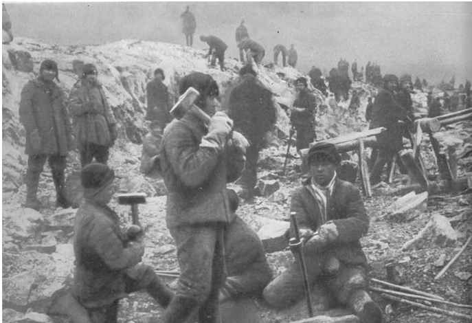
REMOVE THE ROCK. MAKE WAY FOR THE SLUICE!
