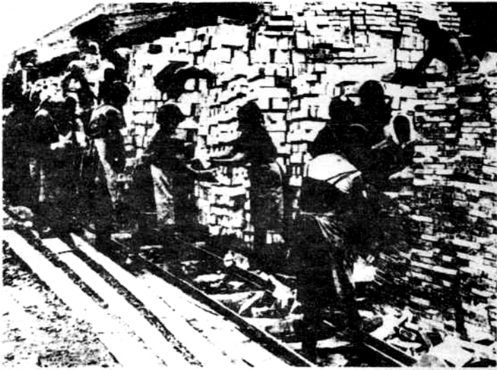
Women sorting bricks—the construction of the first great metallurgical complex at Magnitogorsk, the Urals. (May, 1931)
